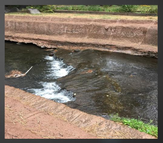
Concrete encased sewer line in Upper Canyon to be rehabilitated and armored
